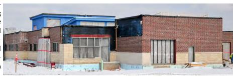
On the police station side, the contractor is completing storm drain piping connections at the roof drains, completing wall framing and laying brick at the sally port. In-wall electrical and plumbing continues, along with the installation of HVAC ductwork and fire sprinkler piping.
